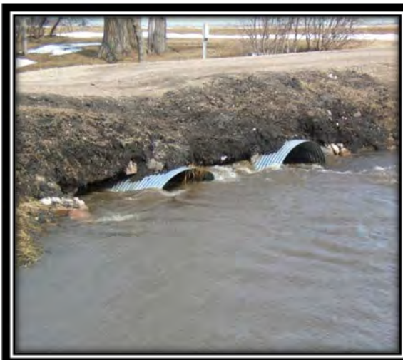
Pipes washing out in Ditch 12
