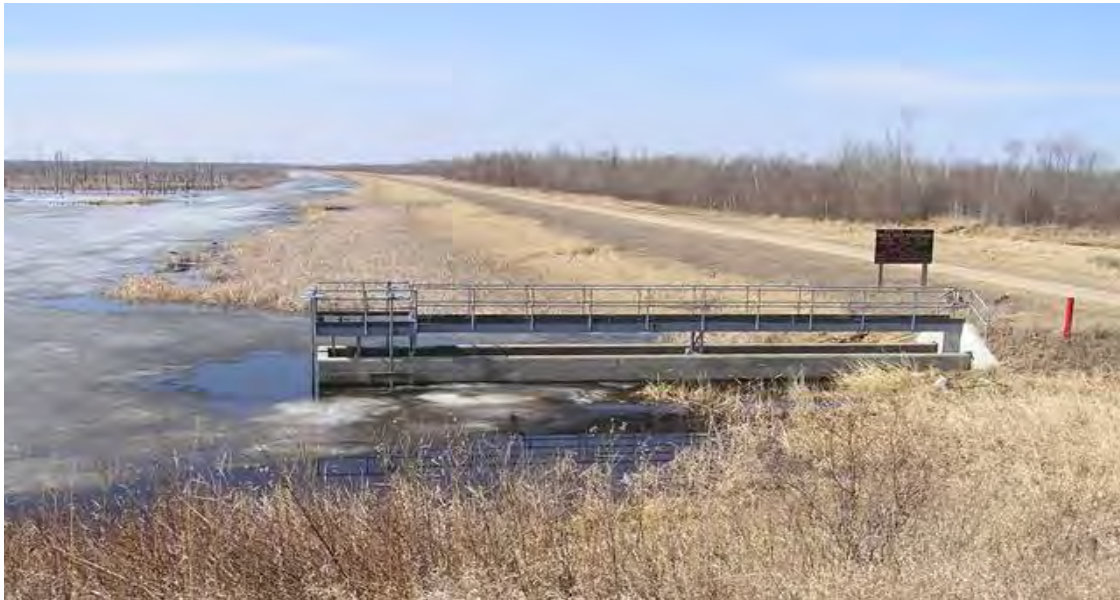
North Pool - Gated Principal Outlet Structure
