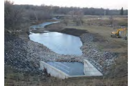
Looking downstream from outlet structure
