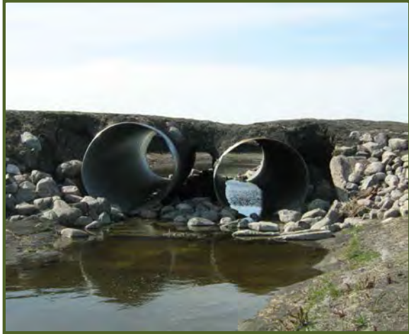
Field road and culvert erosion, Polk County Ditch 53, RLWD Ditch 12, Project No. 169
