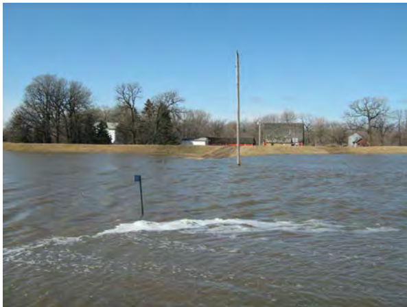
Ring dike protecting farmstead near Red River, Esther Township, Polk County
