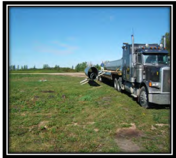
Rolling pipes off the truck
