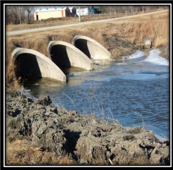
Pipe after cleaning, Section 1, Hammond Township
