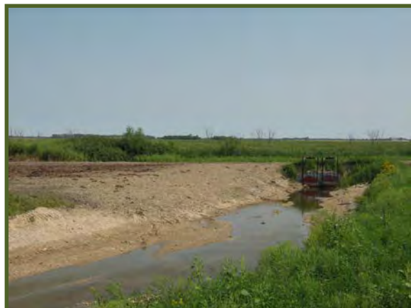
Spring flood erosion near structure between east and west pools, Parnell Impoundment
