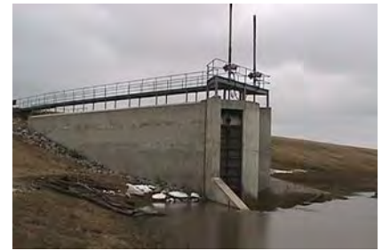
Principal outlet structure hydraulic gate operation
