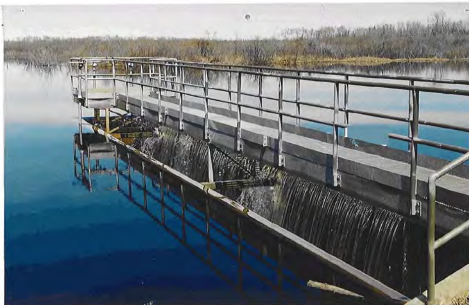
South Pool - Gated Principal Outlet Structure
