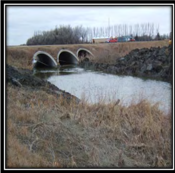
Sediment and willows being removed at the inlet end of pipes in Section 1, Hammond Township
