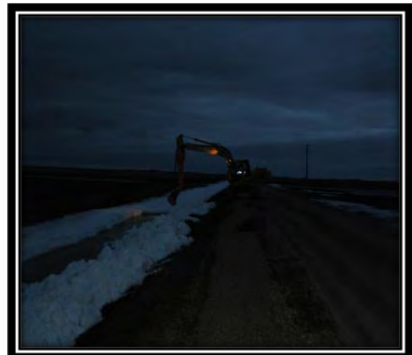
Cleaning snow out of ditch to relieve floodwaters
