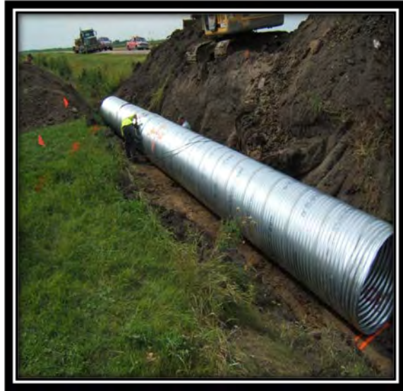
Pipe installation - Branch 1, Ditch 12
