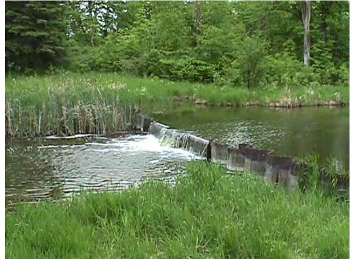
Adjustable stoplog - sheet pile dam
