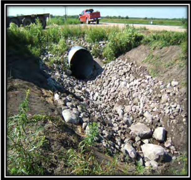
Rock rip rap installed at outlet end of pipe
