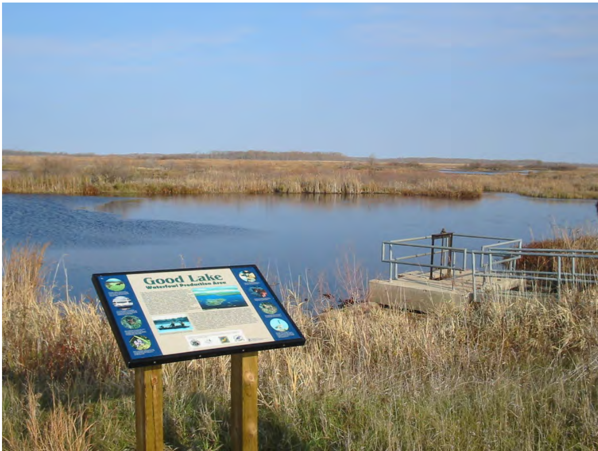
Gated Principal Outlet Structure
