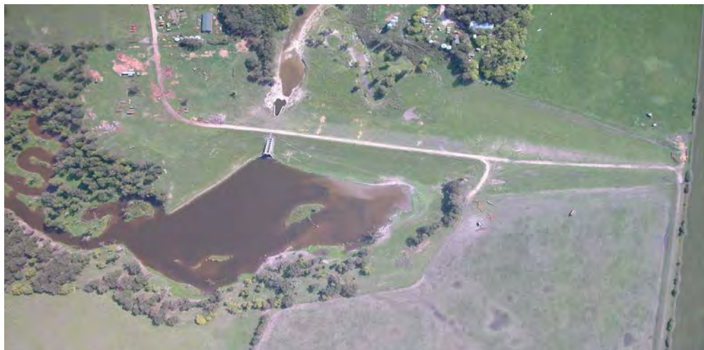
Aerial view of Schirrick Dam looking south
