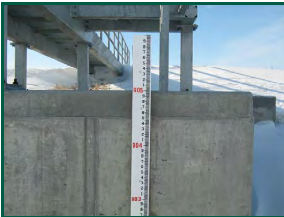
Typical staff gage at structure
