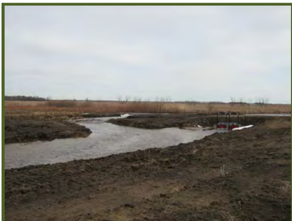
Spring flood erosion near structure between east and west pools, Parnell Impoundment
