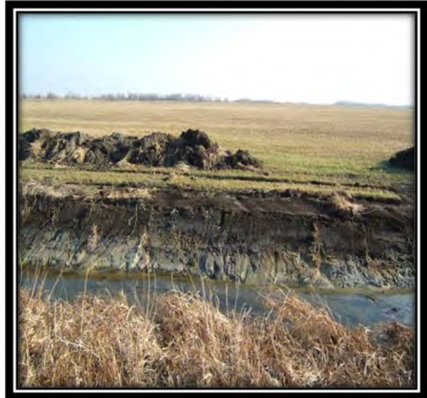
Spoil to be leveled and seeded
