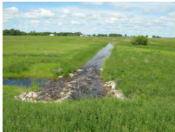
Outlet structure looking west
