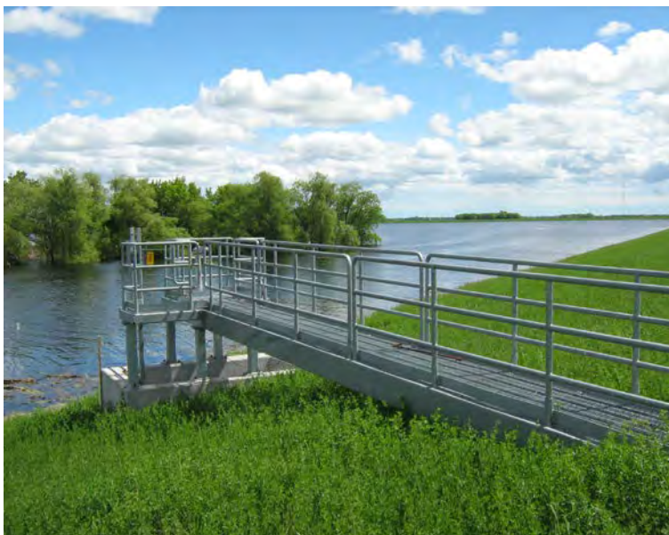
Principal outlet structure
