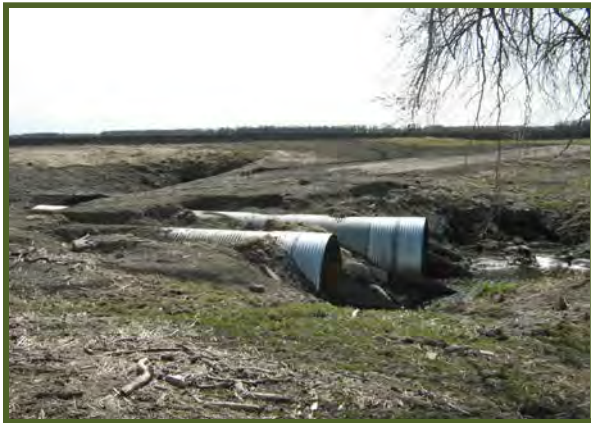
Township road and culverts erosion, Polk County Ditch 53, RLWD Ditch 12, Project No. 169
