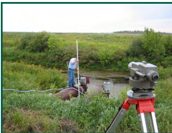
Surveying water lift from river to pump
