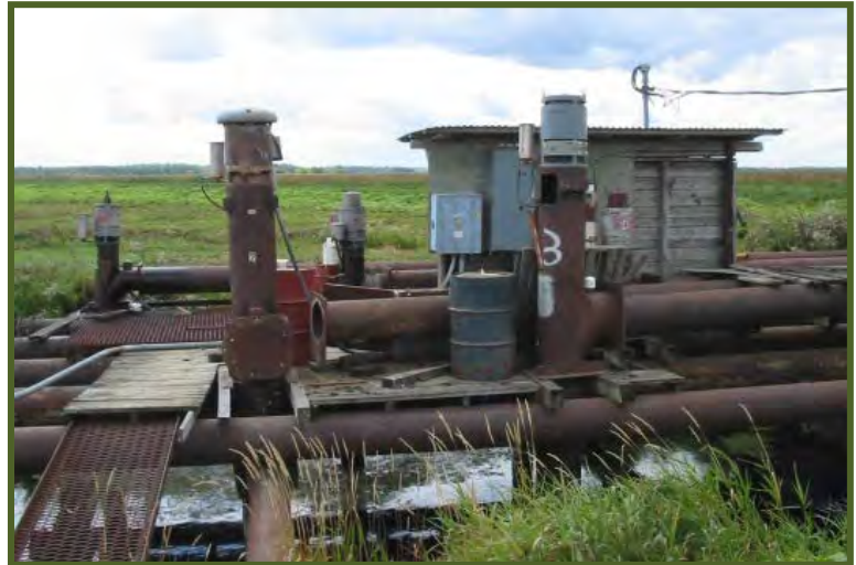
Typical pumping station
