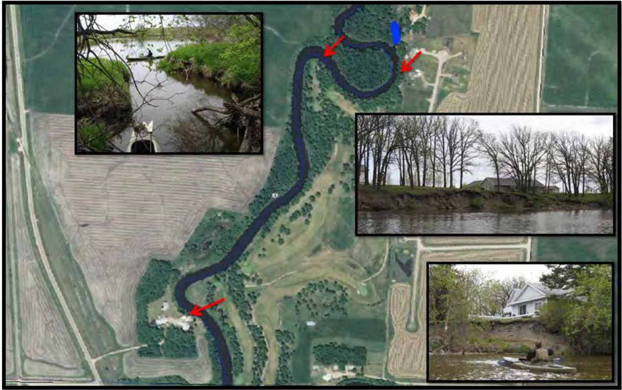
Erosion near the Thief River Golf Club
