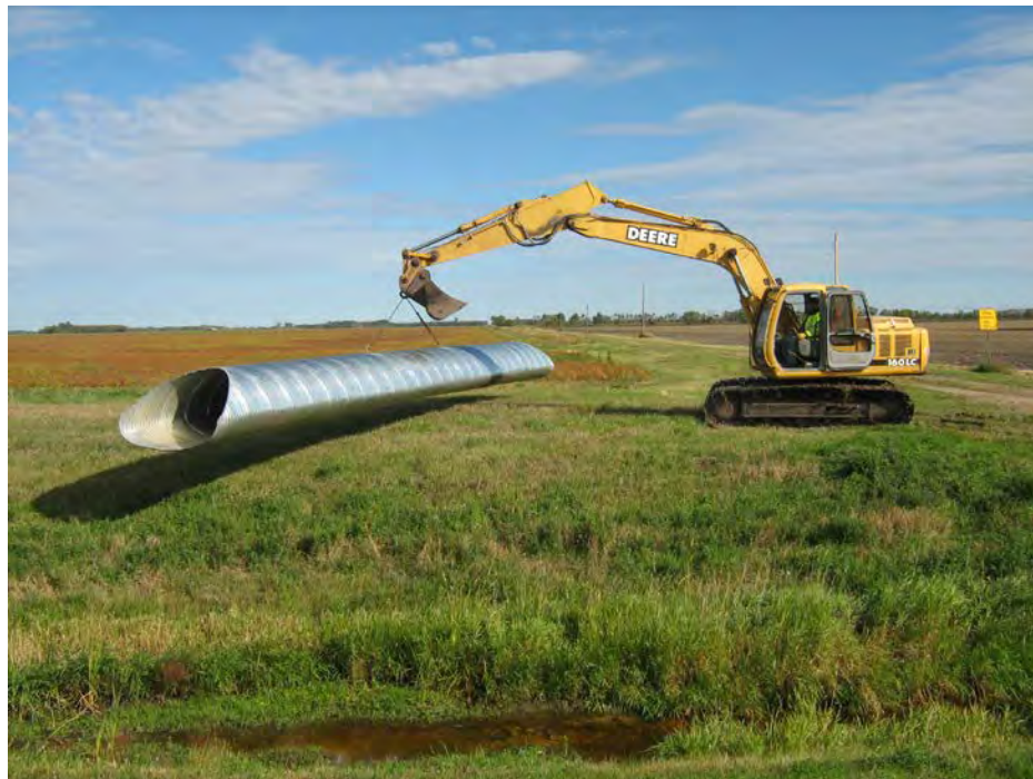
Culvert to be installed in inlet channel of the Euclid East Impoundment
