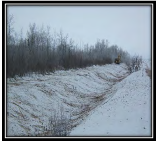
Clearing completed on Ditch 8
