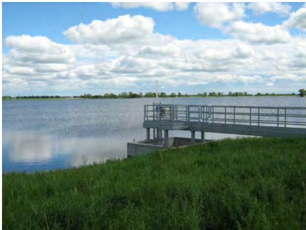
Principal outlet structure
