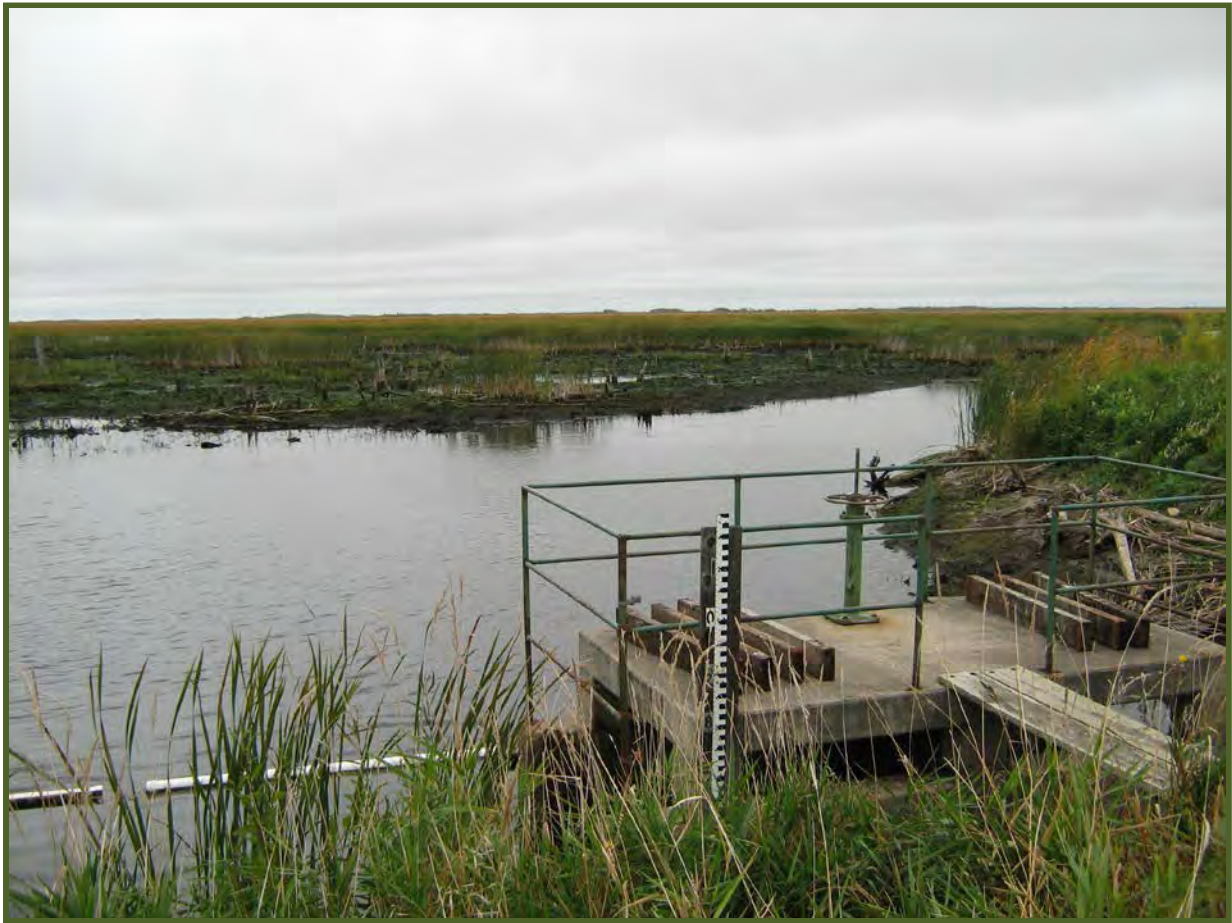
Lost River Pool Outlet Structure
