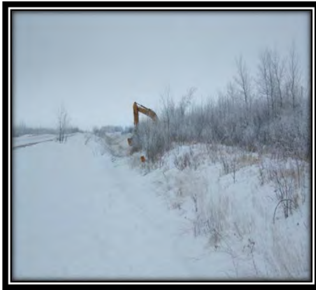
Brushing being done on RLWD 8 Right of Way
